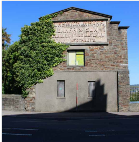
Plate 4: East elevation of the warehouse, looking west (2m scale)
