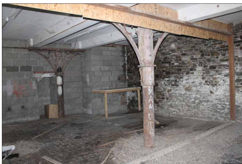
Plate 8: Central ground-floor room of the warehouse, looking southeast
