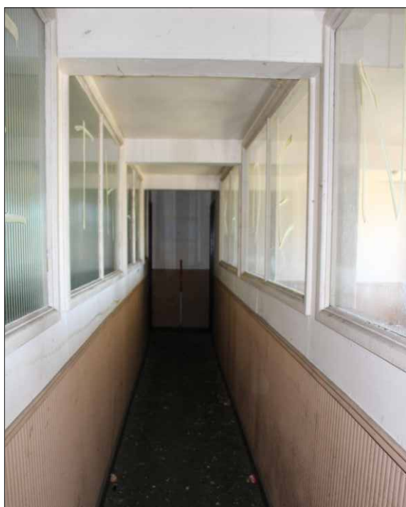
Plate 11: First-floor corridor in the warehouse, looking west (1m scale)
