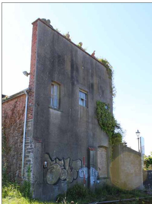
Plate 6: West elevation of the warehouse, looking southeast (2m scale)
