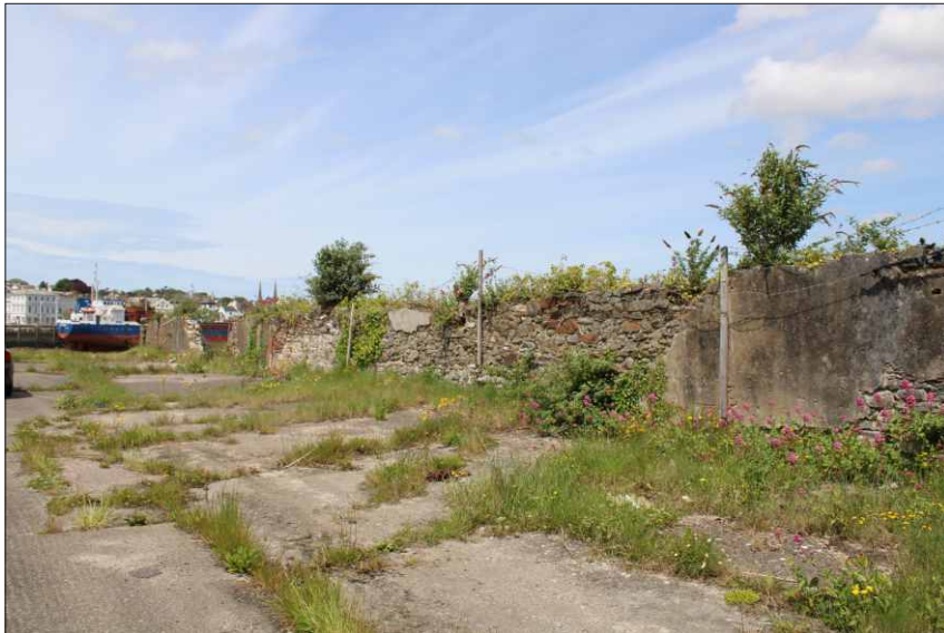
Plate 29: The northern boundary wall of the wharf yard, looking northwest (1m scale)
