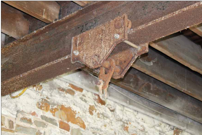
Plate 20: Rolling crane hook on ground floor of the store, looking southeast
