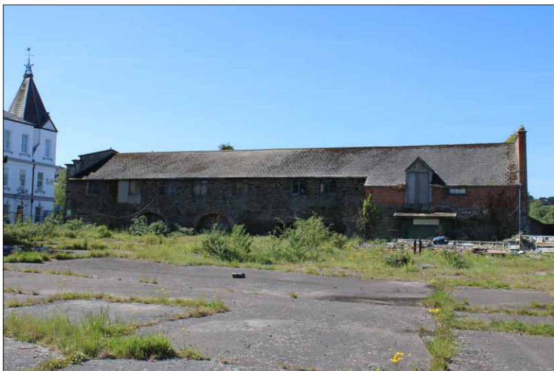
Plate 3: North elevation of the warehouse, looking south (2m scale)
