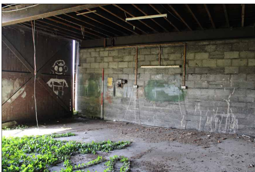
Plate 18: Ground floor of the store (south end), looking northwest (2m scale)
