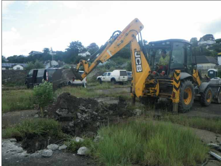
Plate 31: Location of geotechnical test pit 1, work in progress, looking northeast
