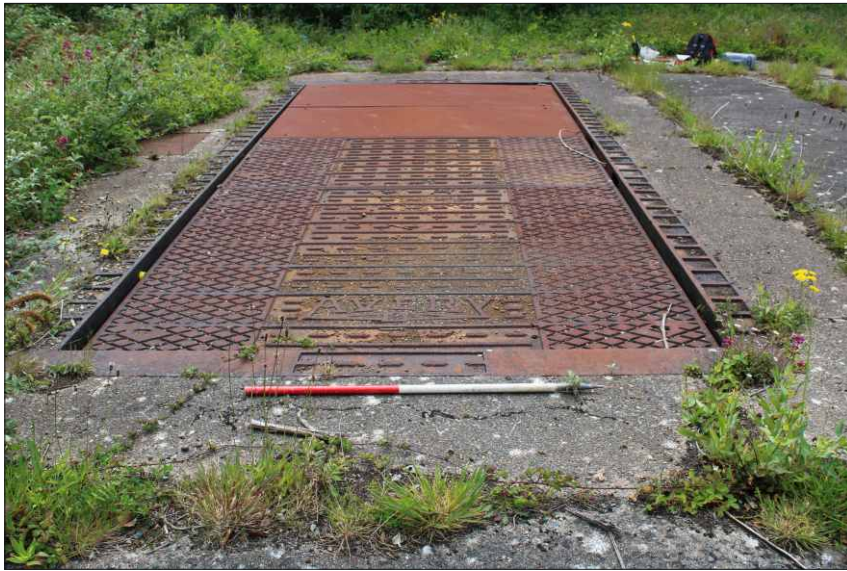
Plate 28: Vehicular weighbridge within the yard, looking south (1m scale)
