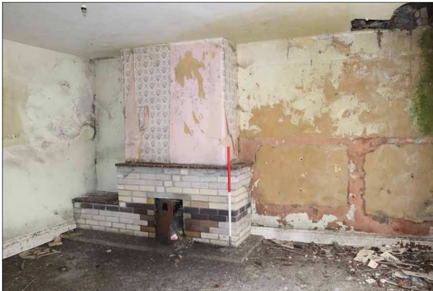
Plate 23: Front reception room in the cottage, looking northwest (1m scale)
