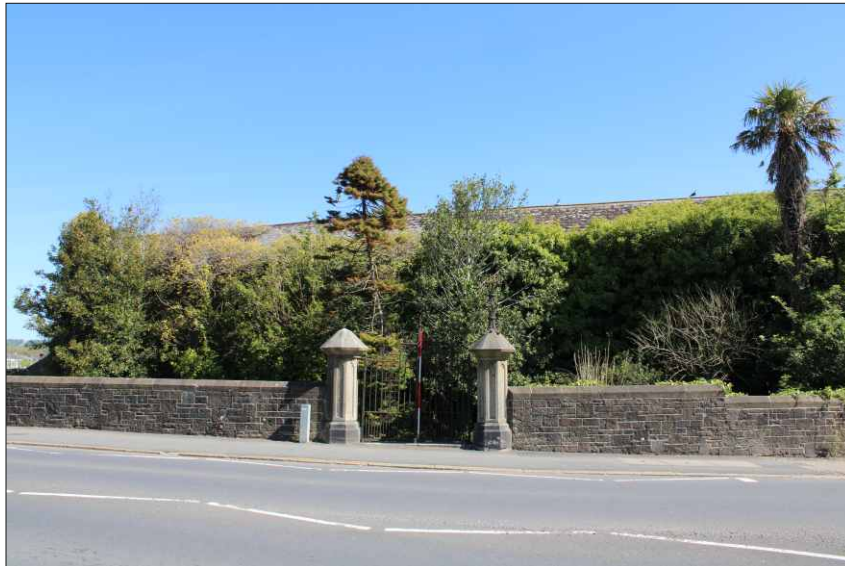
Plate 5: South elevation of the warehouse, looking north (2m scale)
