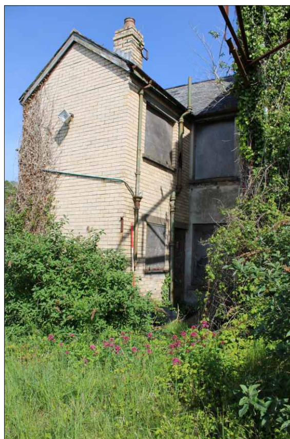
Plate 12: West elevation of the cottage, looking northeast (2m scale)
