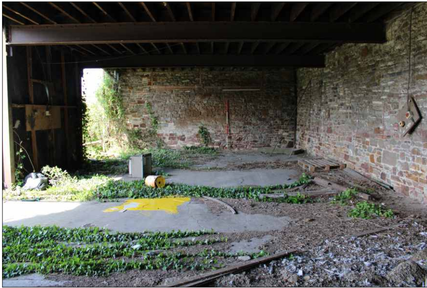
Plate 19: Ground floor of the store (north end), looking north (2m scale)
