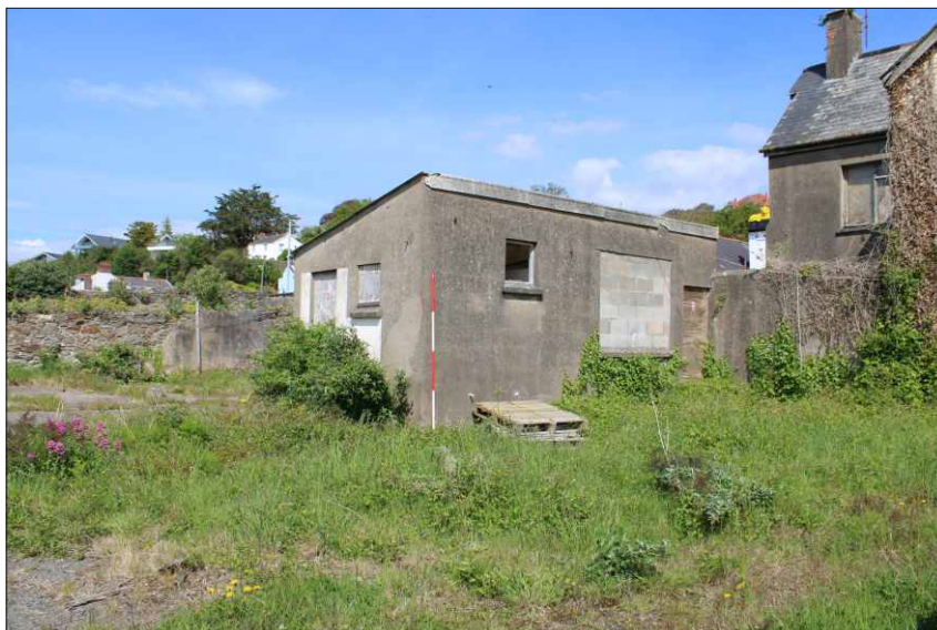
Plate 16: Outbuilding adjacent to cottage, looking northeast (2m scale)
