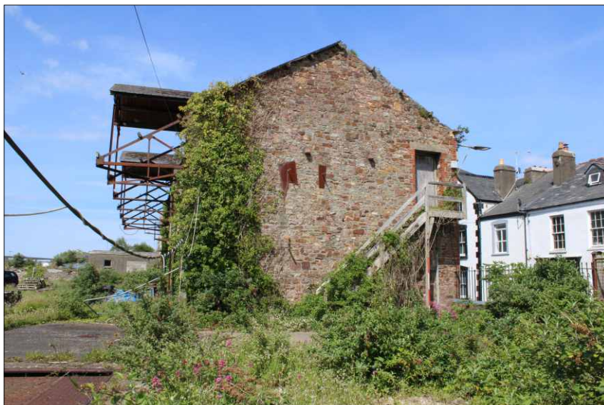
Plate 15: South elevation of the store, looking north (2m scale)
