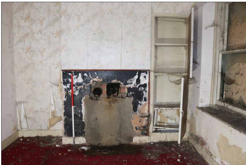
Plate 24: Fireplace in the kitchen of the cottage, looking south (1m scale)
