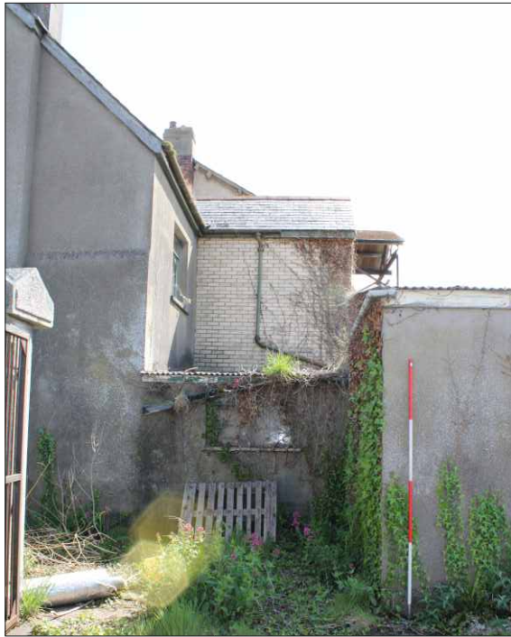
Plate 13: North elevation of the cottage showing the extension, looking south (2m scale)
