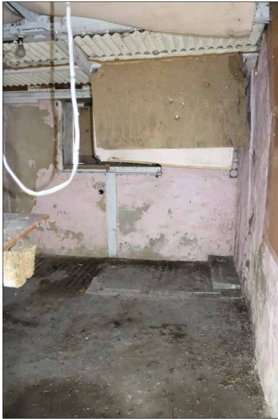
Plate 25: North extension of the cottage, looking north
